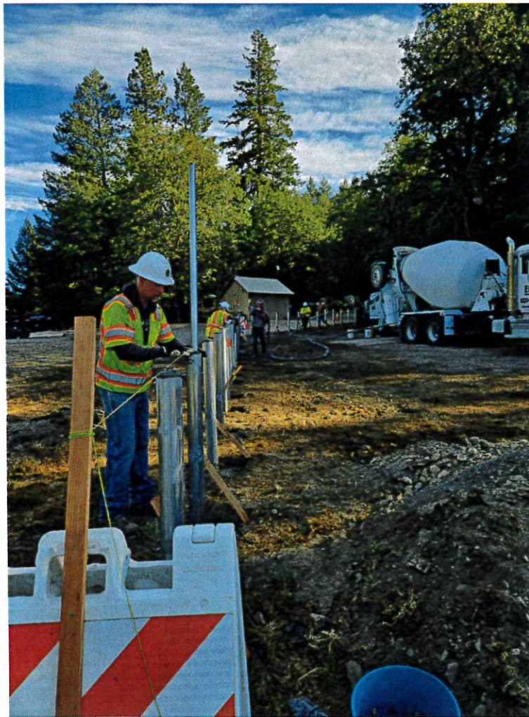
District staff installing bollards At Ruth Rec
