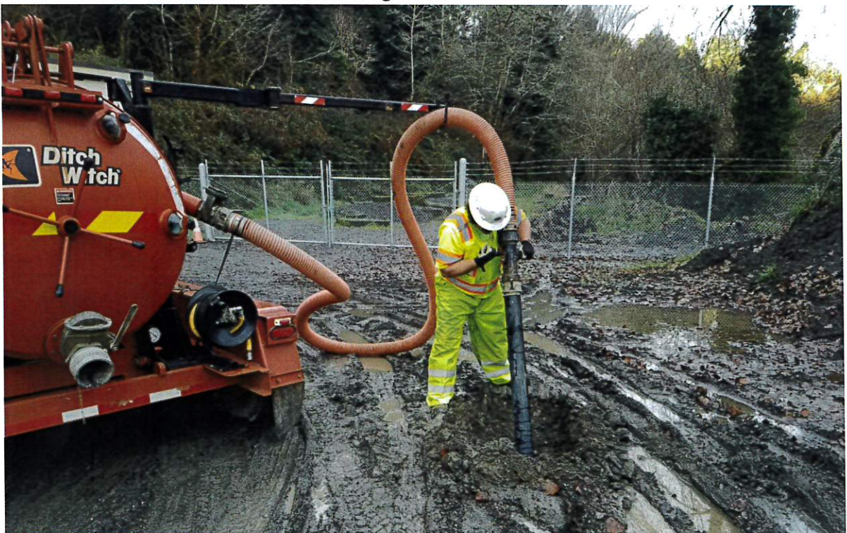
Boom deployed during operation, notice how it supports the vacuum line above the operator.
