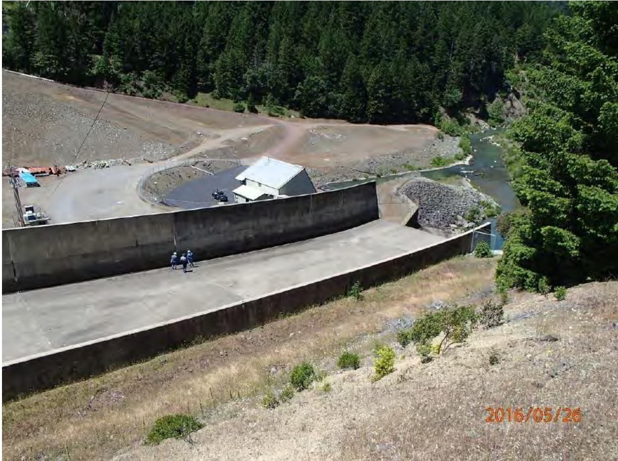
Photo 4 - Lower End of Spillway
