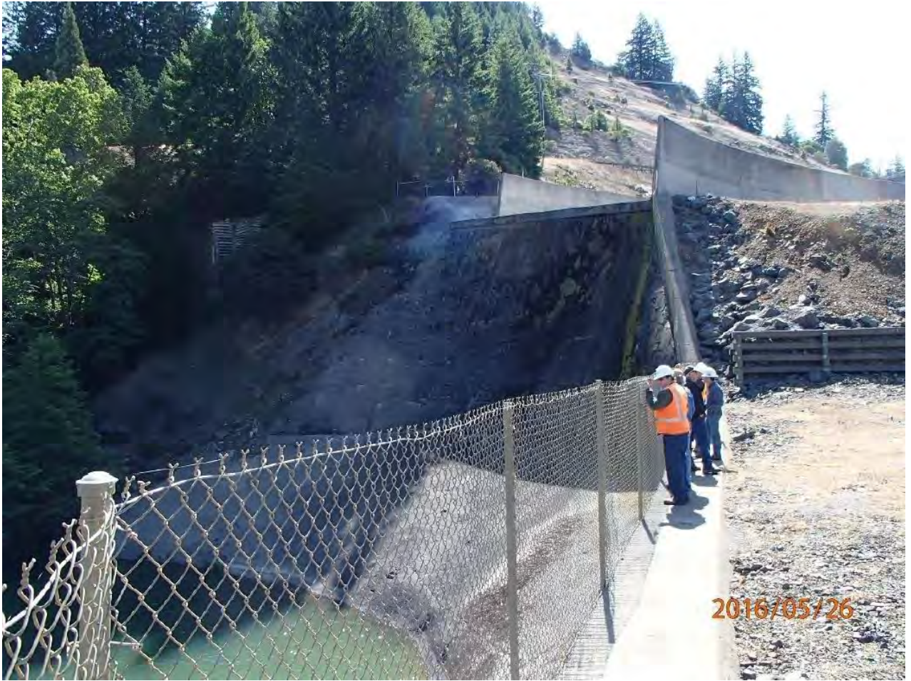
Photo 5 - End of Flip Bucket of Spillway
