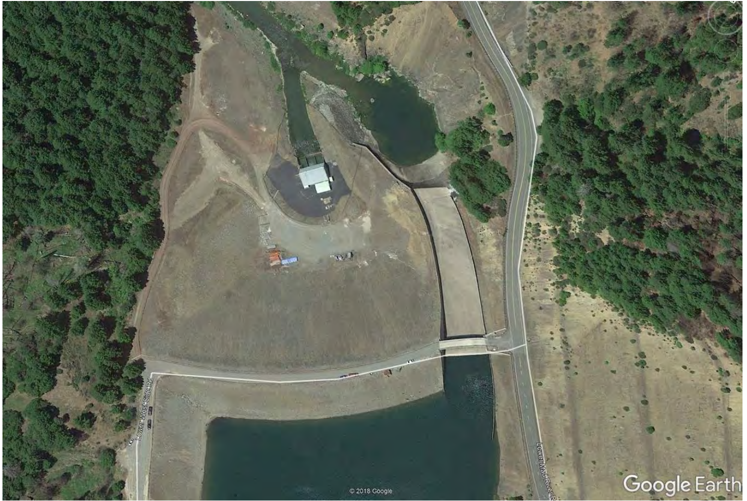
Photo 1 - Overview of R.W. Matthews Dam
