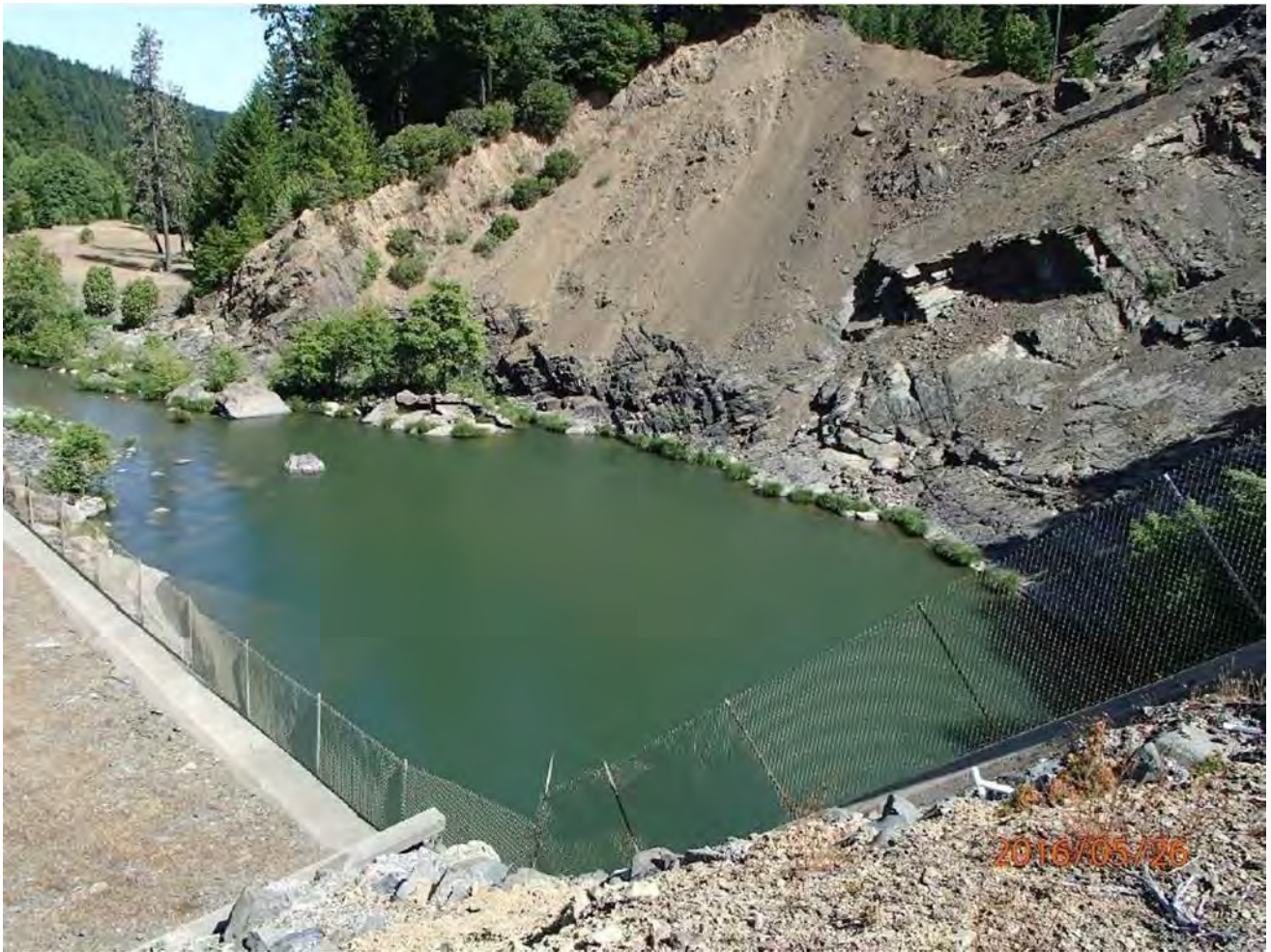
Photo 6 - Spillway Plunge Pool
