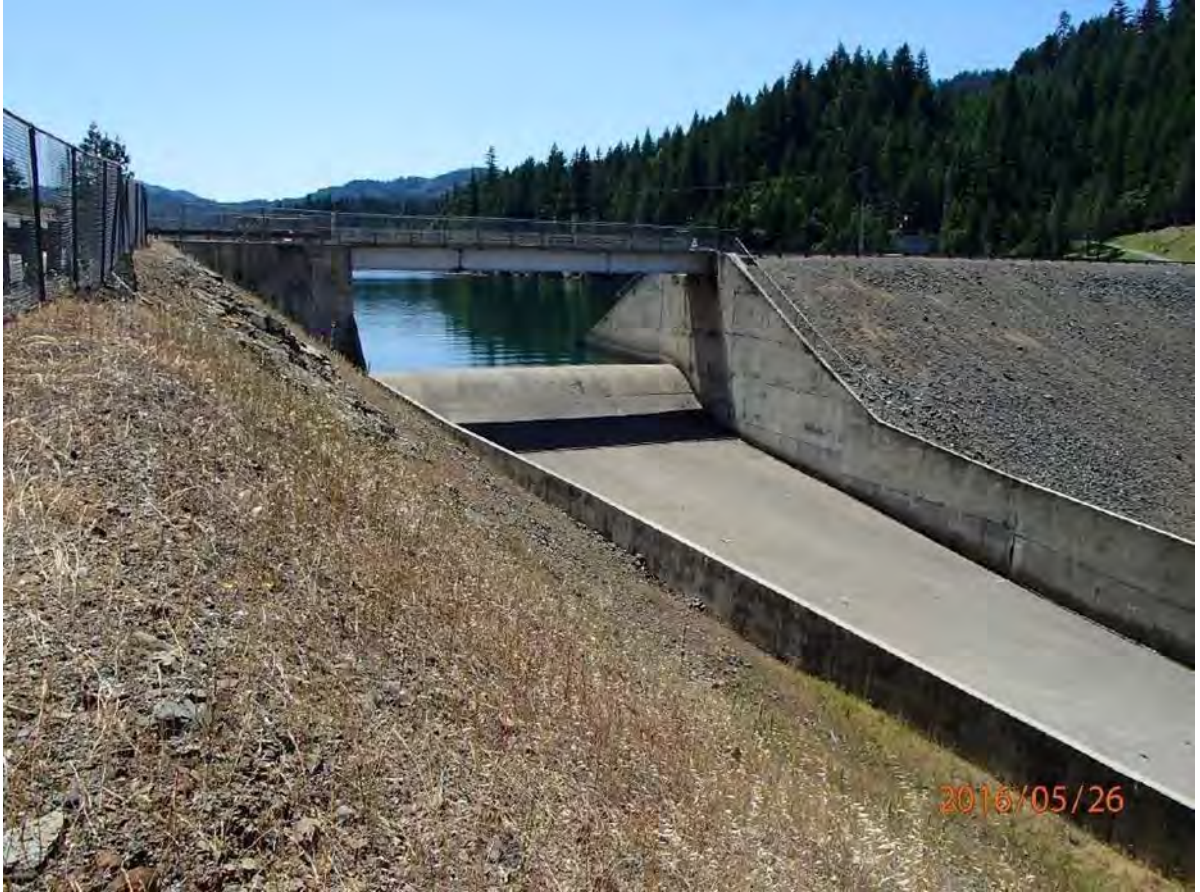
Photo 3 - Upper End of Spillway
