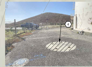
3 EXISTING VAULT AND VALVE - DEMOLITION PHOTO
